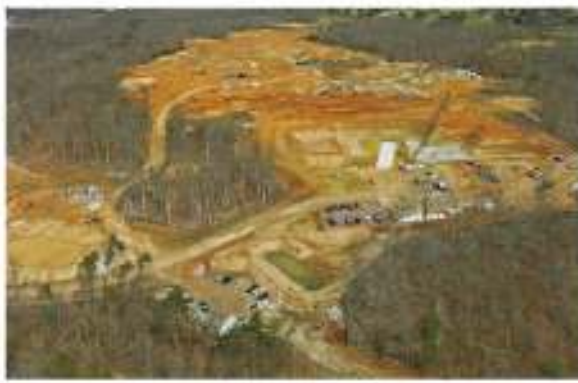
Aerial photo of the National Army Museum construction site in March, 2017
